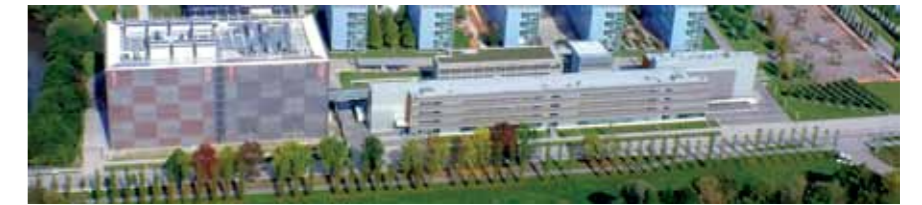
Figure 6: The LRZ building after the extension 2009-2011 in Garching near Munich.
