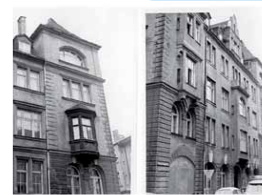
Figure 4: The first LRZ building.
